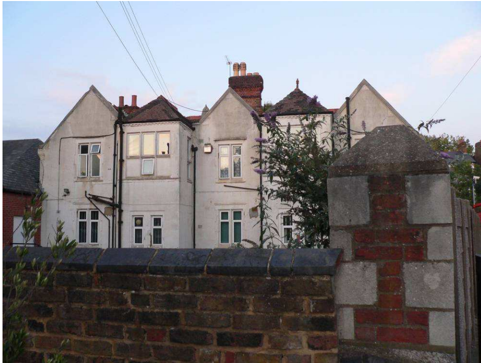
Boone's Almshouses, south range rear elevation, seen from Lampmead Road, October 2011
